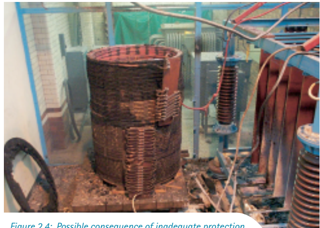
Figure 2.4: Possible consequence of inadequate protection
